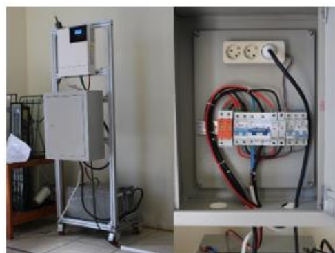
Gambar 7. Instalasi Panel Kontrol
